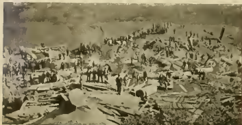
EXPLOSION OF TWENTY-SEVEN BOILERS ON A TRAIL OF THIRTY-TWO AT HENRY CLAY COLLEGE, SHAWANK, PA., DECEMBER 11, 1894.
